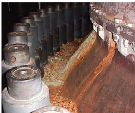
This is what inspectors ignored.
