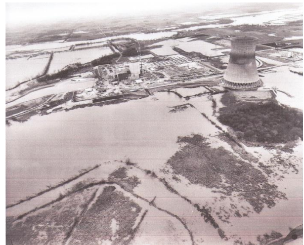
Davis-Besse construction site floods in 1972.
